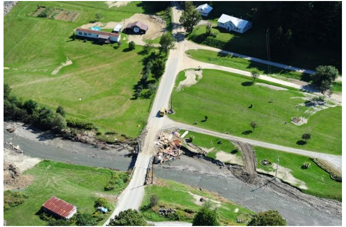
In Bridgewater Corners a house washed up against the bridge, blocking water and threatening to wipe out the bridge. Photo by Mansfield Heliflight.
