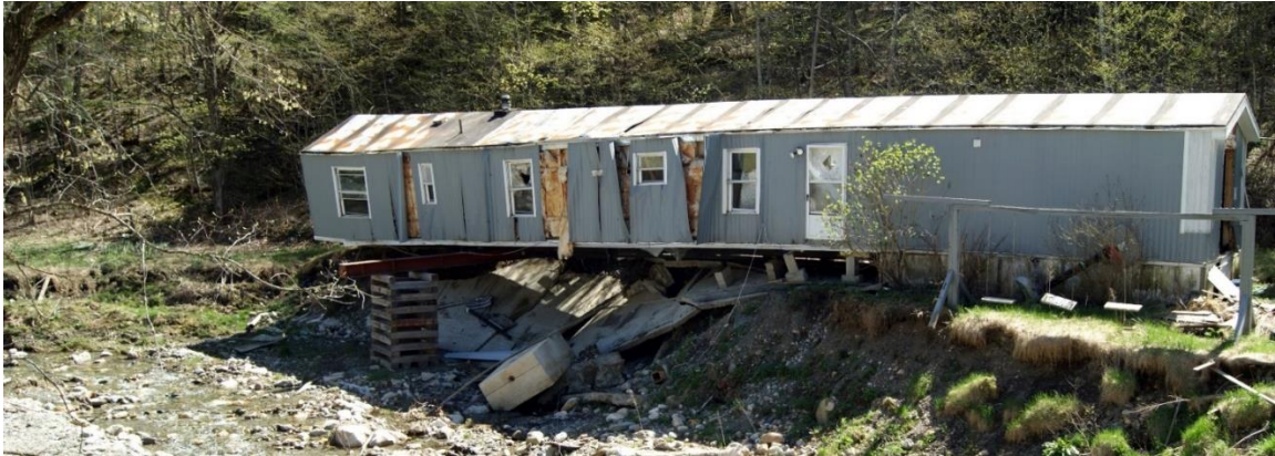
Structures built in floodplains like this one along the Danby-Pawlet Road are a risk for homeowners and the community at large. Floods can threaten to wash them downstream into bridges or other structures. Photo by Lori Fisher.
