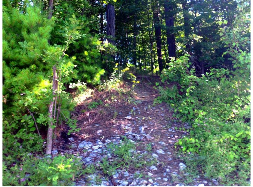
Failure to provide controlled access to the waterfront can lead to development of herd paths like this one. Once a herd path forms, erosion accelerates along it and it is extremely difficult to reestablish vegetation. Photo by Mike Winslow.
